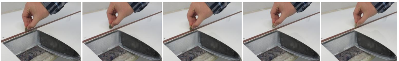
Fig. 3 – coin tap test along main wall position
