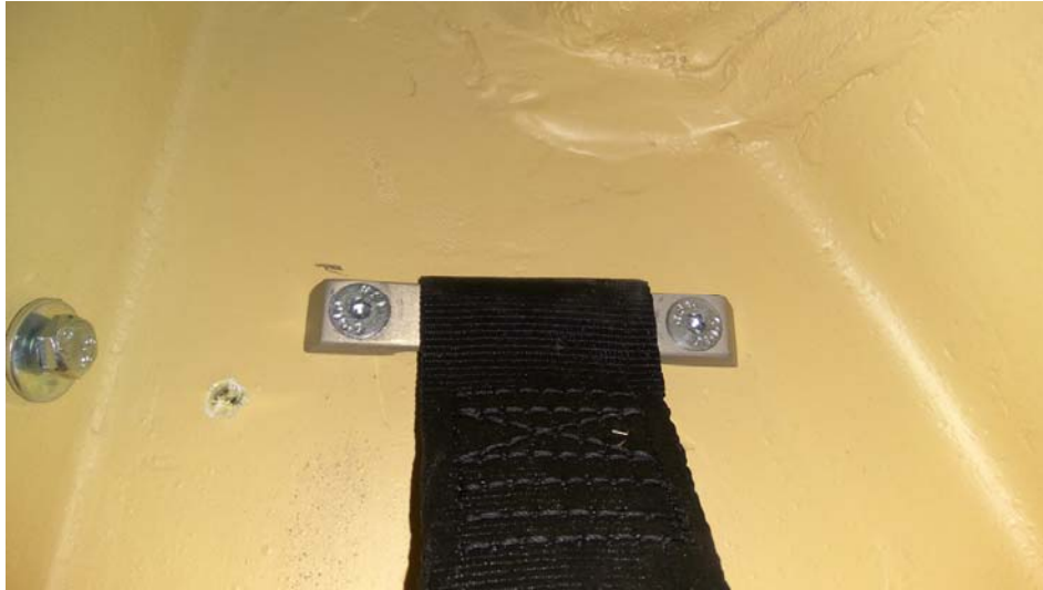
Fig. 3-3-1-2 (View from cabin)
